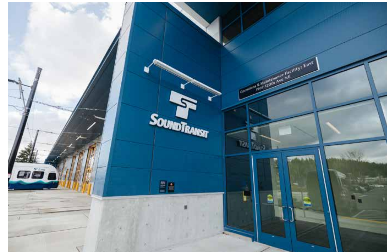
The Entrance of the Operations and Maintenance Facility: East in Bellevue.
