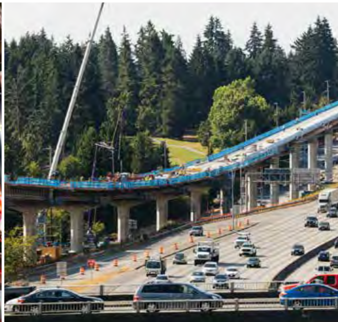
Moving forward: beginning major construction on Lynnwood Link extension.
