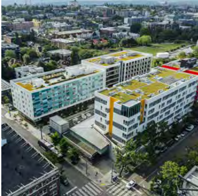
Helping create affordable housing: breaking ground and partnering with Amazon.
